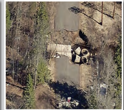
Post-flood damage assessment.
