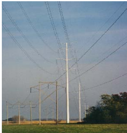
High Voltage Transmission Lines
